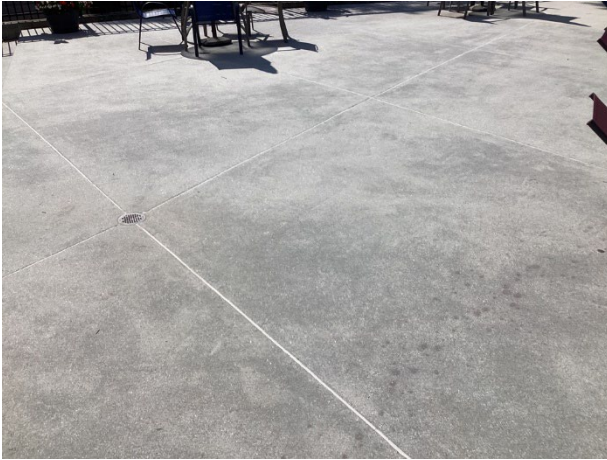
Concrete pool deck overview
