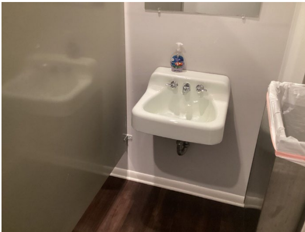
Rest room fixtures
