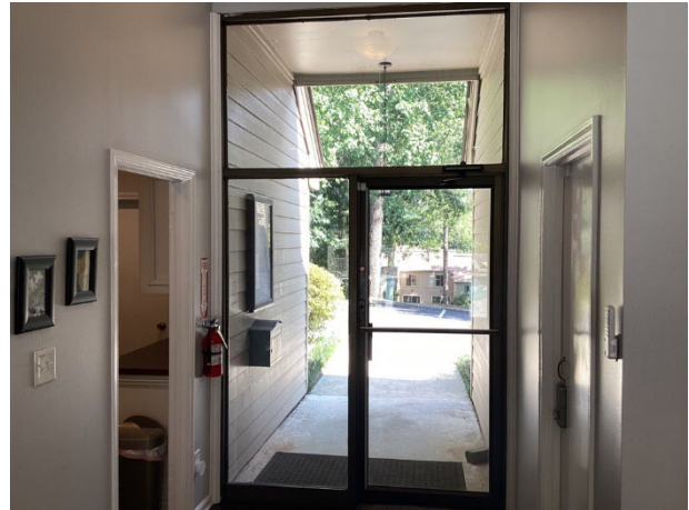
Hinged doors and fixed windows
