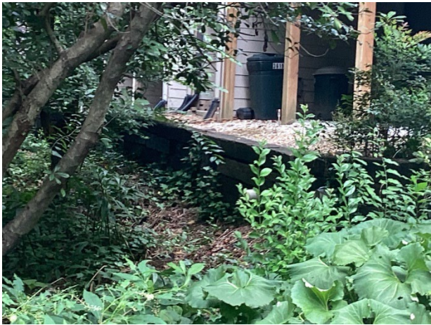
Timber retaining wall overview
