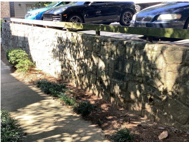
Stone retaining wall
