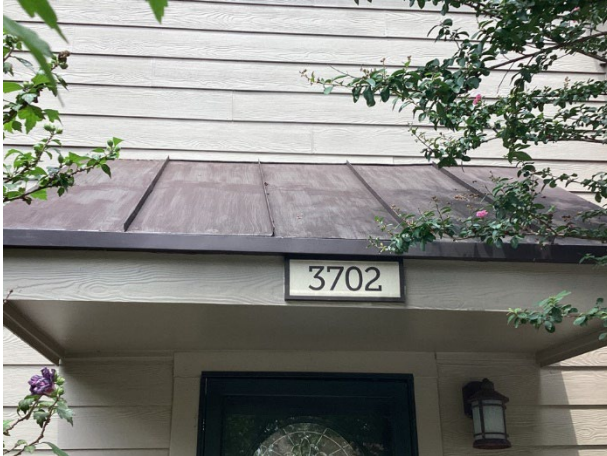
Metal roof at townhouse
