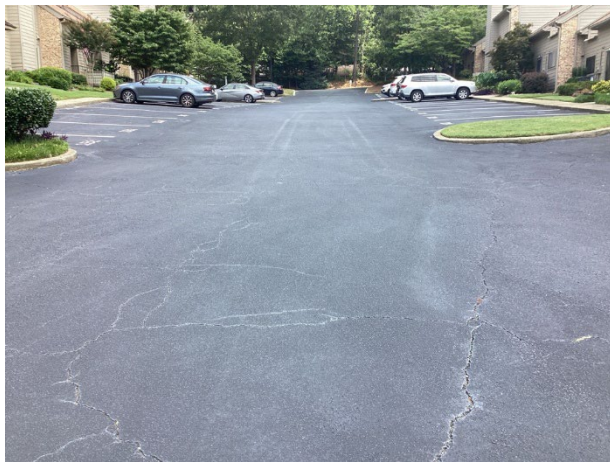
Parking area pavement overview
