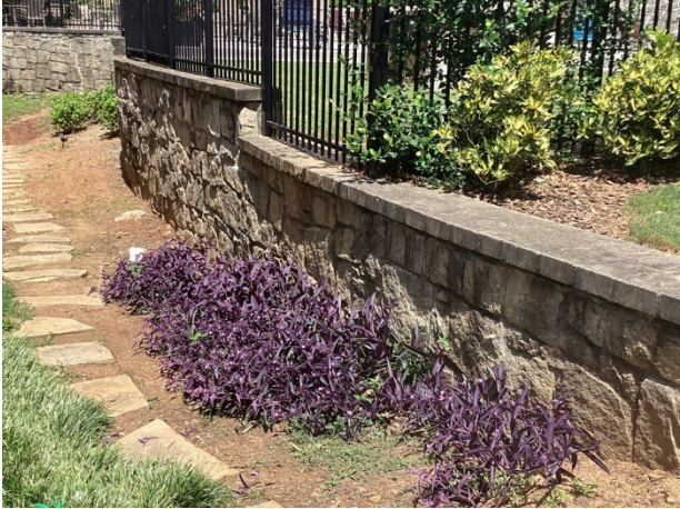
Stone retaining wall at pool
