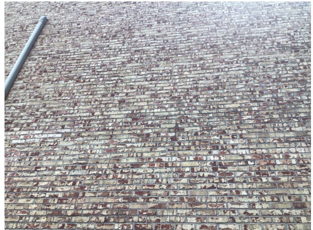
Masonry walls overview
