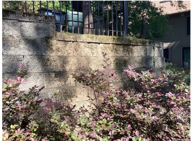
Masonry retaining wall
