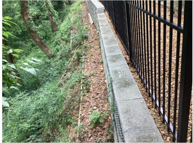
Masonry retaining wall
