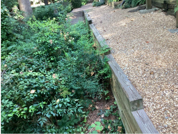
Timber retaining wall overview
