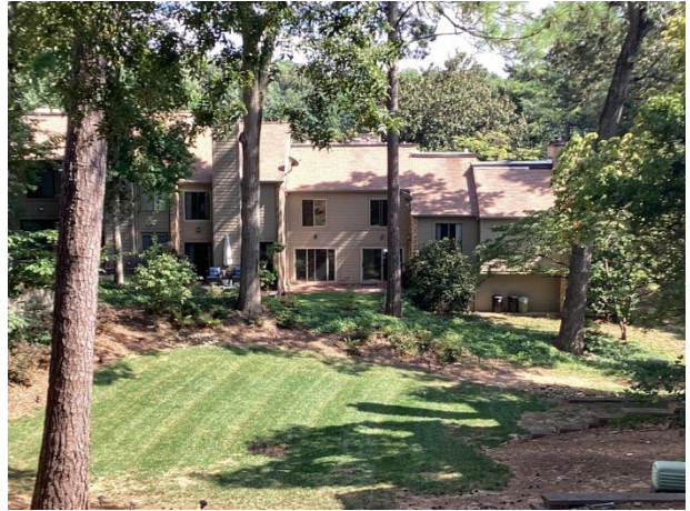
Townhome exterior overview
