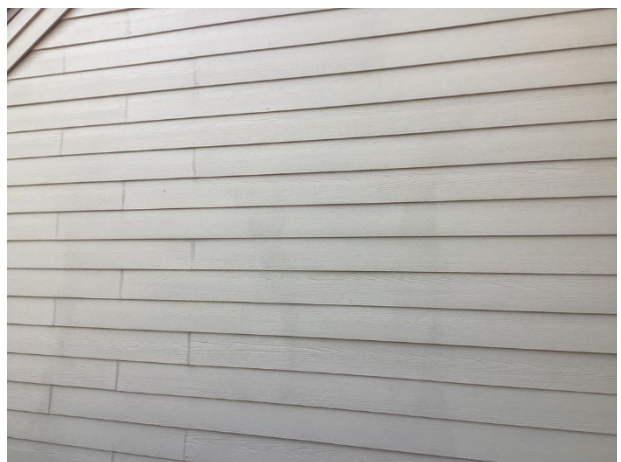
Fiber cement siding overview
