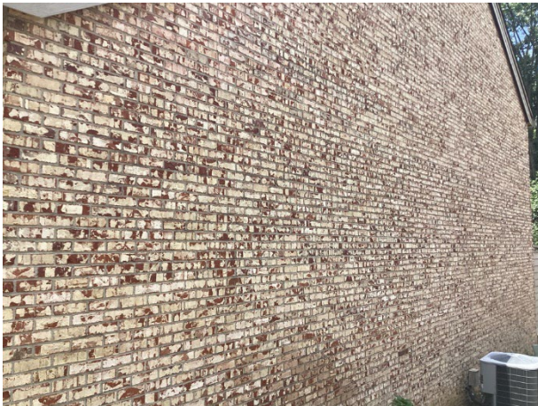
Masonry walls overview
