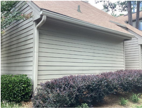
Aluminum gutters and downspouts at clubhouse
