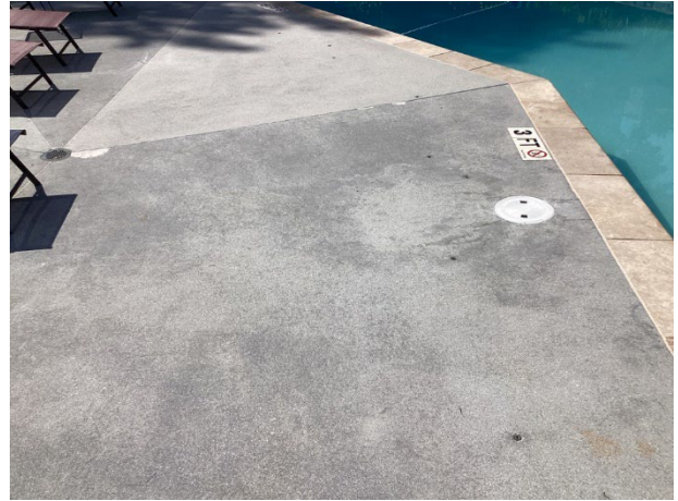
Concrete pool deck overview
