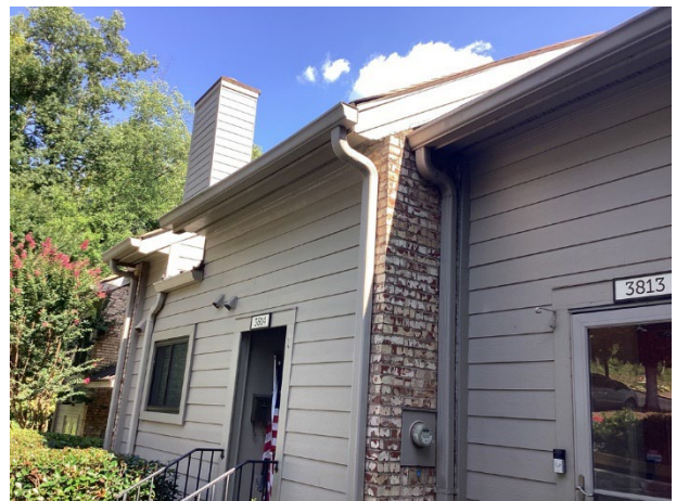
Aluminum gutters and downspouts
