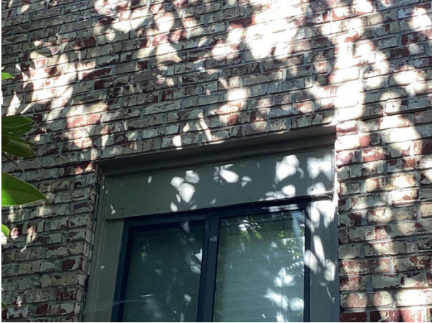
Masonry walls overview
