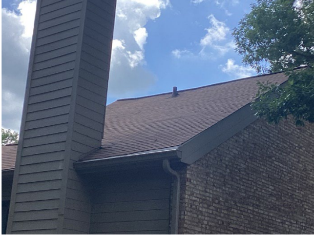
Townhome roof overview
