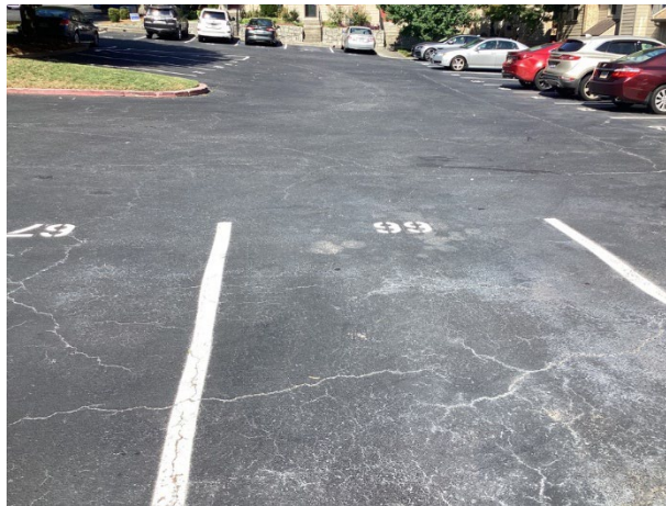
Parking area pavement overview
