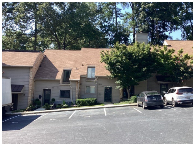
Townhome exterior overview
