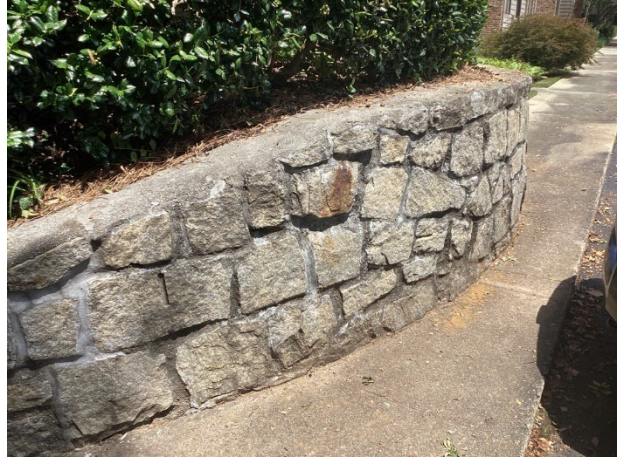
Stone retaining wall
