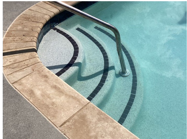
Pool plaster overview
