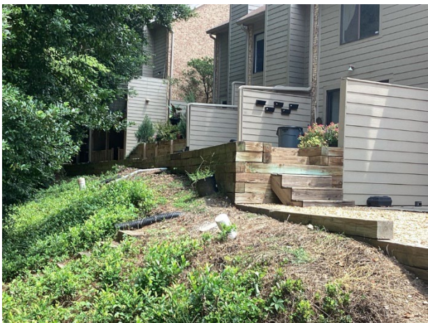
Timber retaining wall overview
