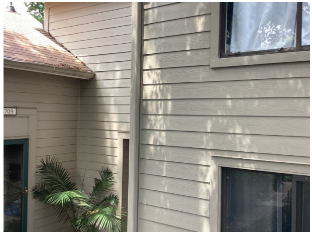
Fiber cement siding overview
