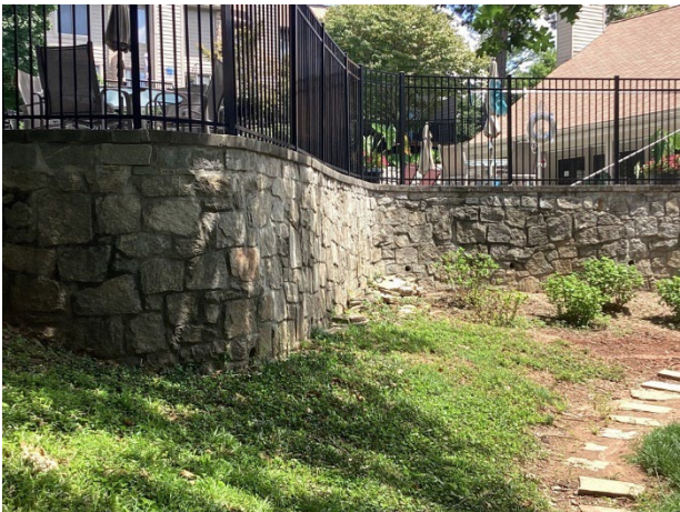
Stone retaining wall at pool
