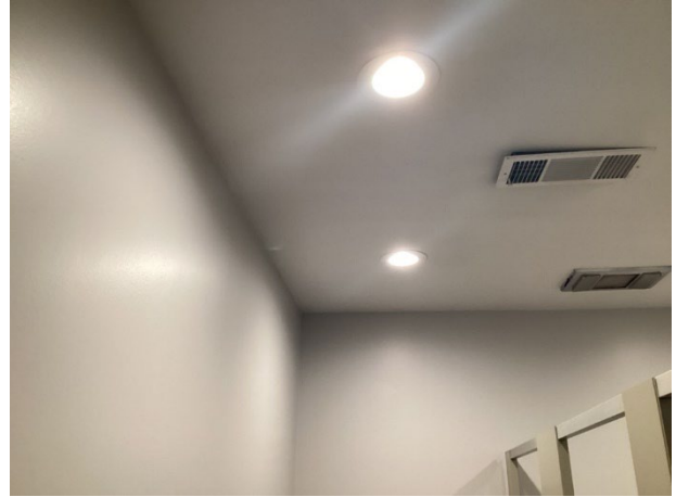
Paint finish and light fixtures overview
