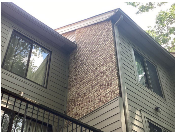
Masonry walls overview
