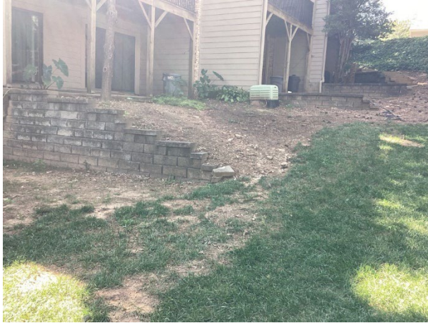
Masonry retaining walls overview
