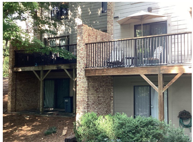
Masonry walls overview
