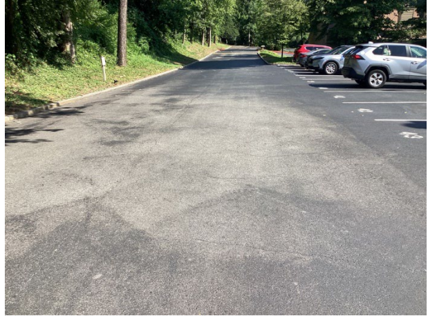
Stonewall Dr pavement overview
