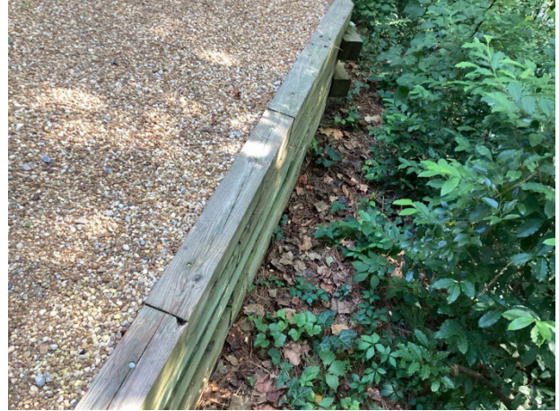
Timber retaining wall overview
