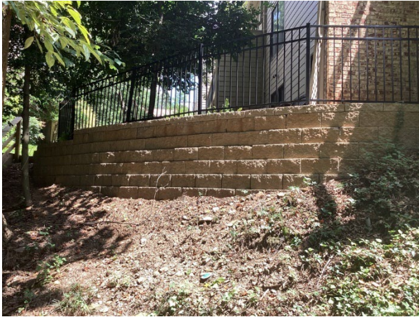
Masonry retaining wall
