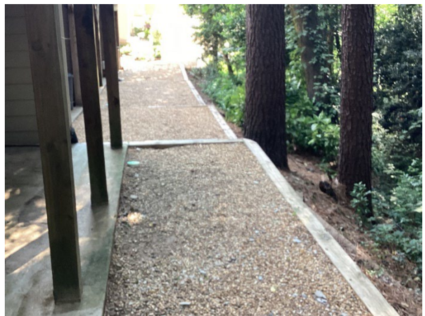
Timber retaining wall overview
